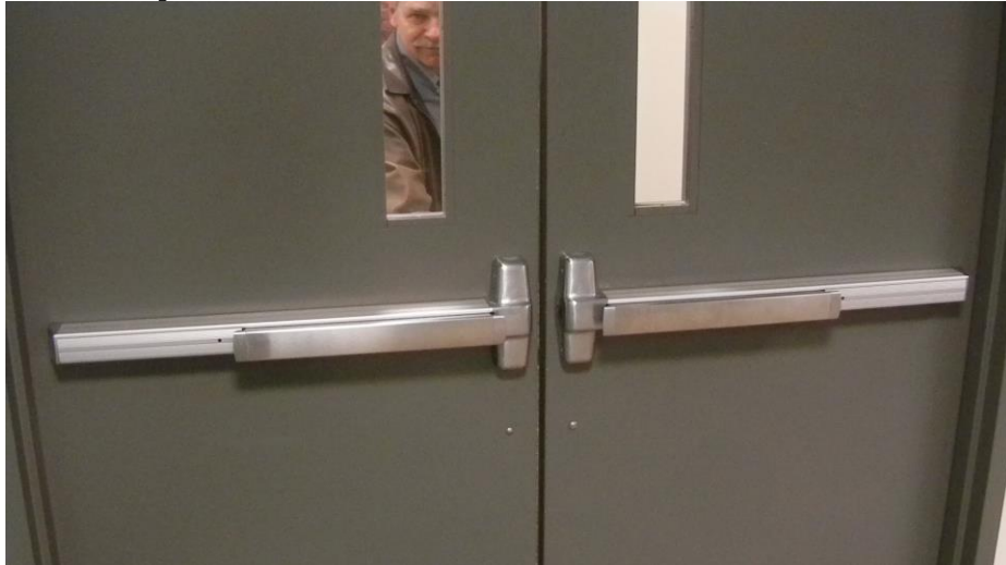
Typical double doors
